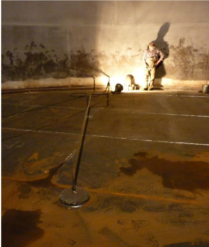
Measuring line to tank centre
